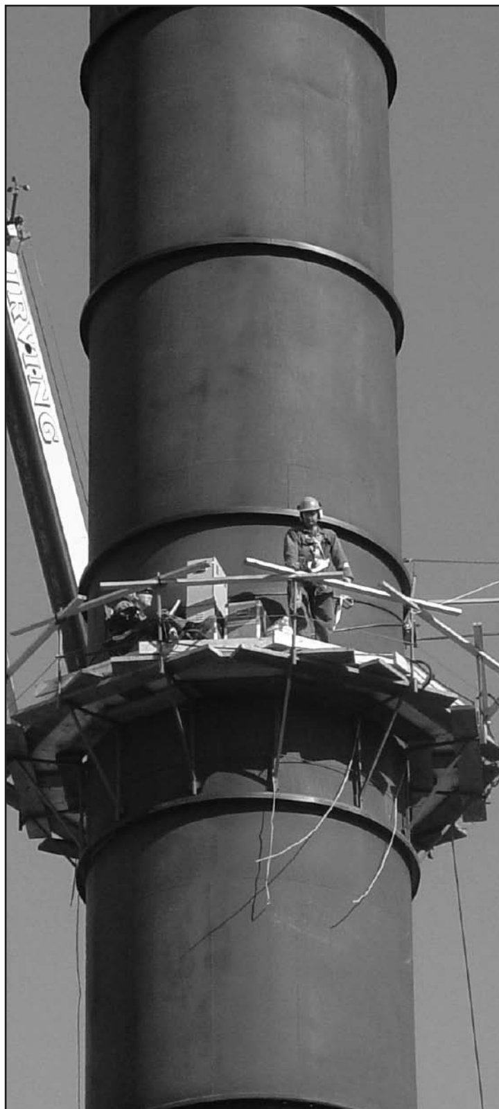
Jacques Whitford test stack emissions on the #3 Crude Unit.
