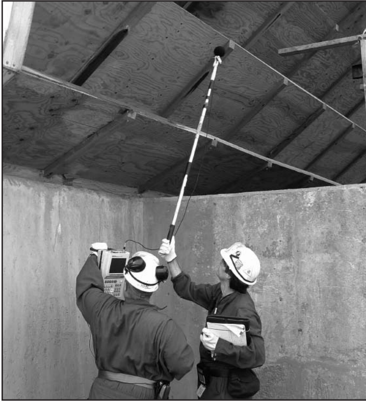
HGC Engineering performs sound surveying on one of the cooling towers.
